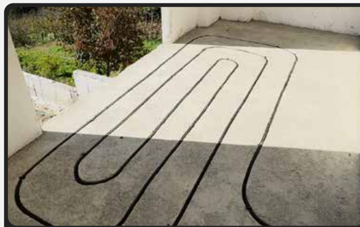
Ağacık / Sakarya | With Screed Applied FloorFlex Installation
