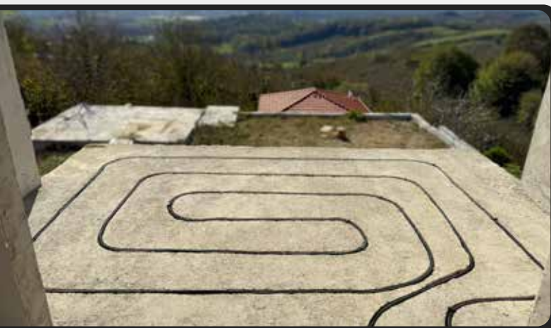
Ağacık / Sakarya | With Screed Applied FloorFlex Installation
