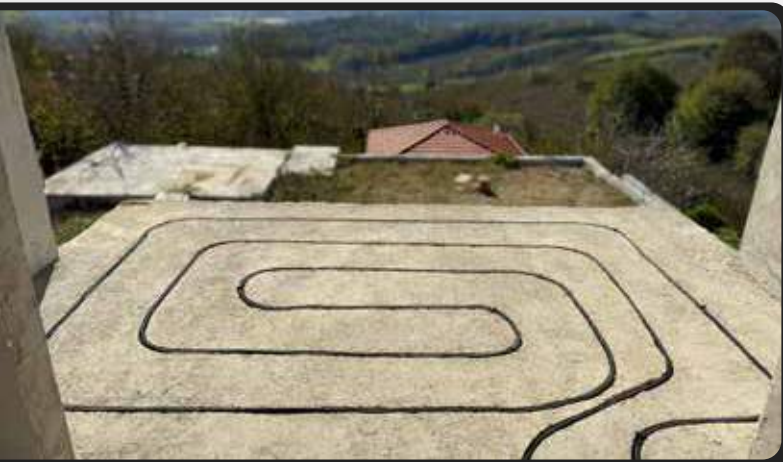
Ağacık / Sakarya | With Screed Applied FloorFlex Installation
