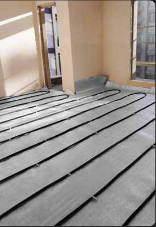
Cevizli / İstanbul | With Insulation FloorFlex Installation Mat Applied
