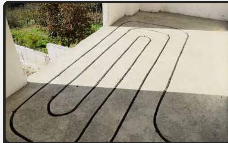
Ağacık / Sakarya | With Screed Applied FloorFlex Installation
