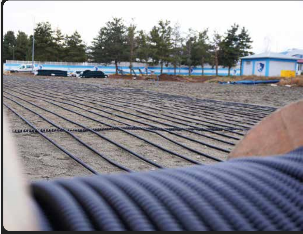
Yakutiye / Erzurum FloorFlex Installation
